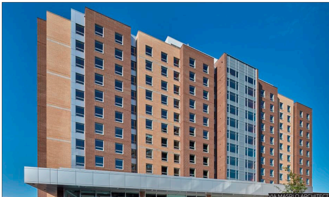
VIA MASRI O ARCHITECTS
