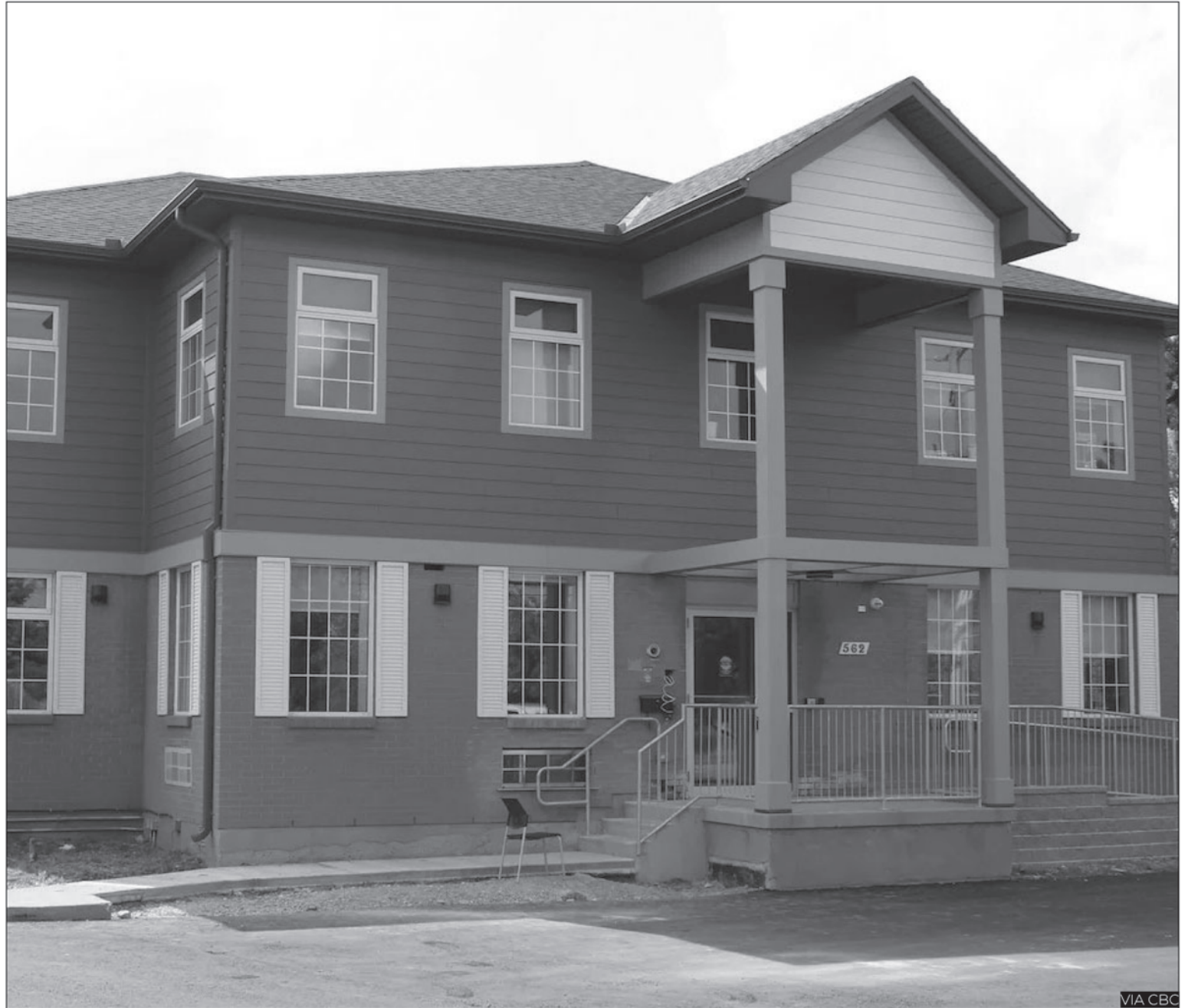
The House of Friendship received $100,000 to support addictions and substance use treatment services.
