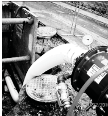
CIPP liner being installed.
