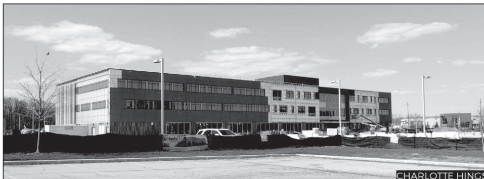
Outside view of Evolv1 building in progress (May 2018)
